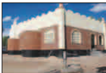
Masajid, Classroom Blocks & Borehole Construction
